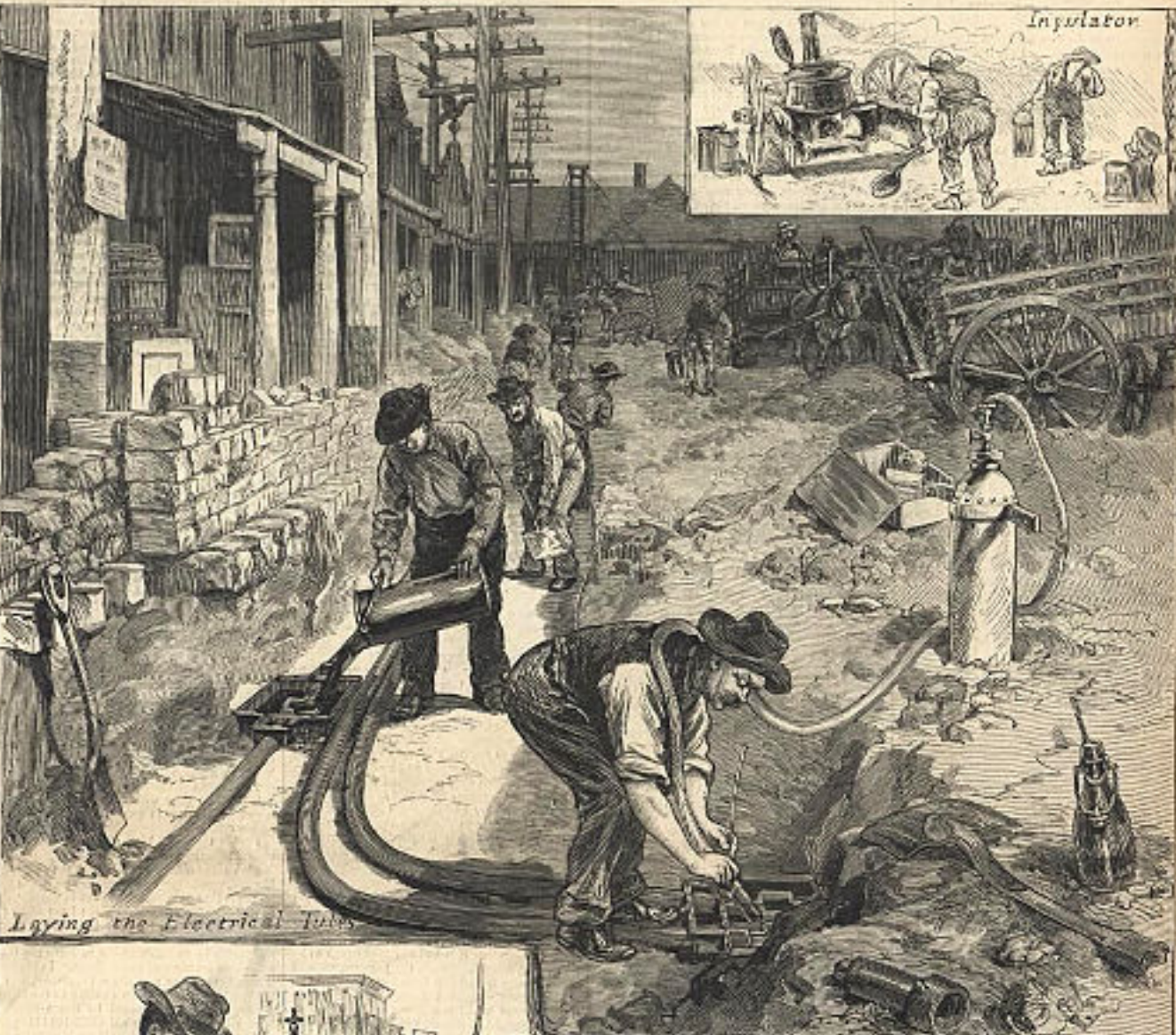
The Electric Light in Houses — Laying the tubes for wires in the streets of New York," by W. P. Snyder for Harpers Weekly, June 24, 1882
